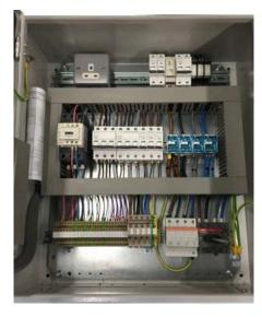
Final connections within the panel should be completed by the commissioning engineer during commissioning of the unit.
