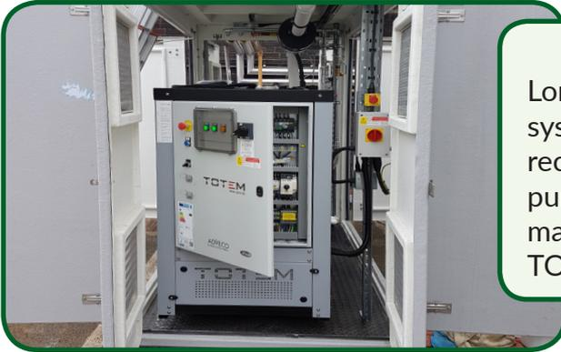
London Fire Brigade invested in an onsite cogeneration system from Adveco for electricity production and recovered heat. The TOTEM T10 was housed in a small purpose built Packaged Plant Room. To allow for regular maintenance the plant room provides full access to the TOTEM m-CHP unit.
