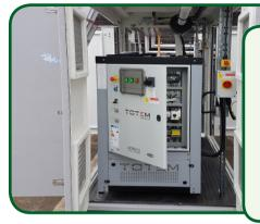
London Fire Brigade's Chelsea station invested in an onsite cogeneration system from Adveco for electricity production and recovered heat. The TOTEM T10 was housed in a small purpose built packaged plant room located in space to the building's rear. To allow for regular maintenance the plant room provides access on all four sides to the TOTEM m-CHP unit.
