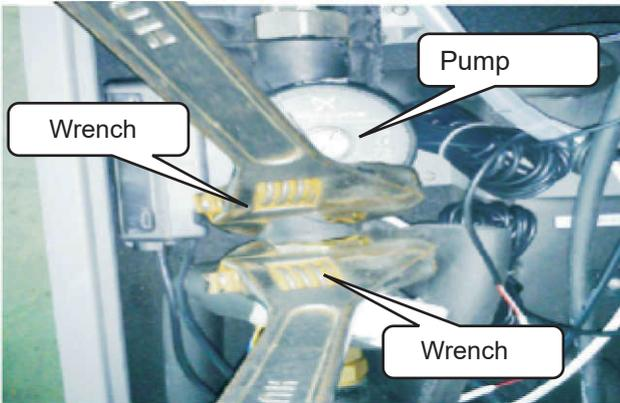
Figure 9-4 Pump disassembly
