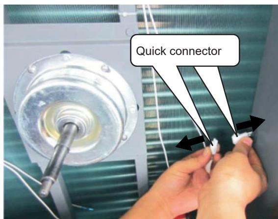
Figure 9-17 Disconnect the quick connector
