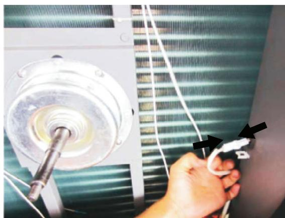
Figure 9-18 Connect the new wire heater
