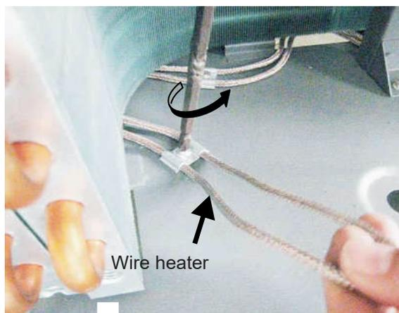
Figure 9-16 Bottom wire heater
