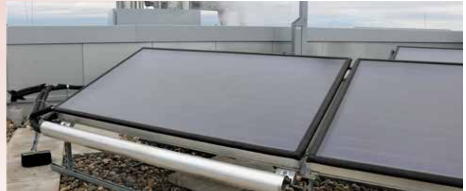
| Solar thermal preheat for gas-fired water heating
