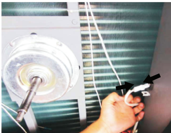
Figure 9-17 Connect the new wire heater
