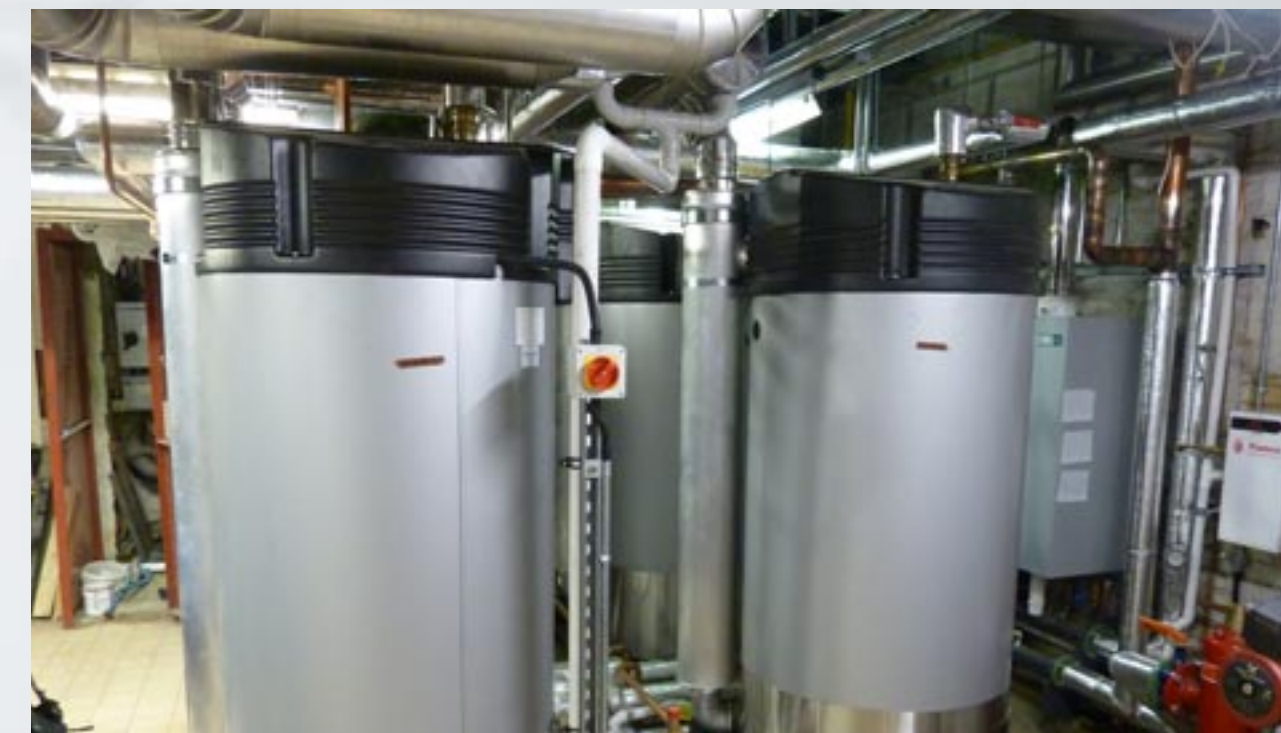
Solar thermal plant installed in basement
