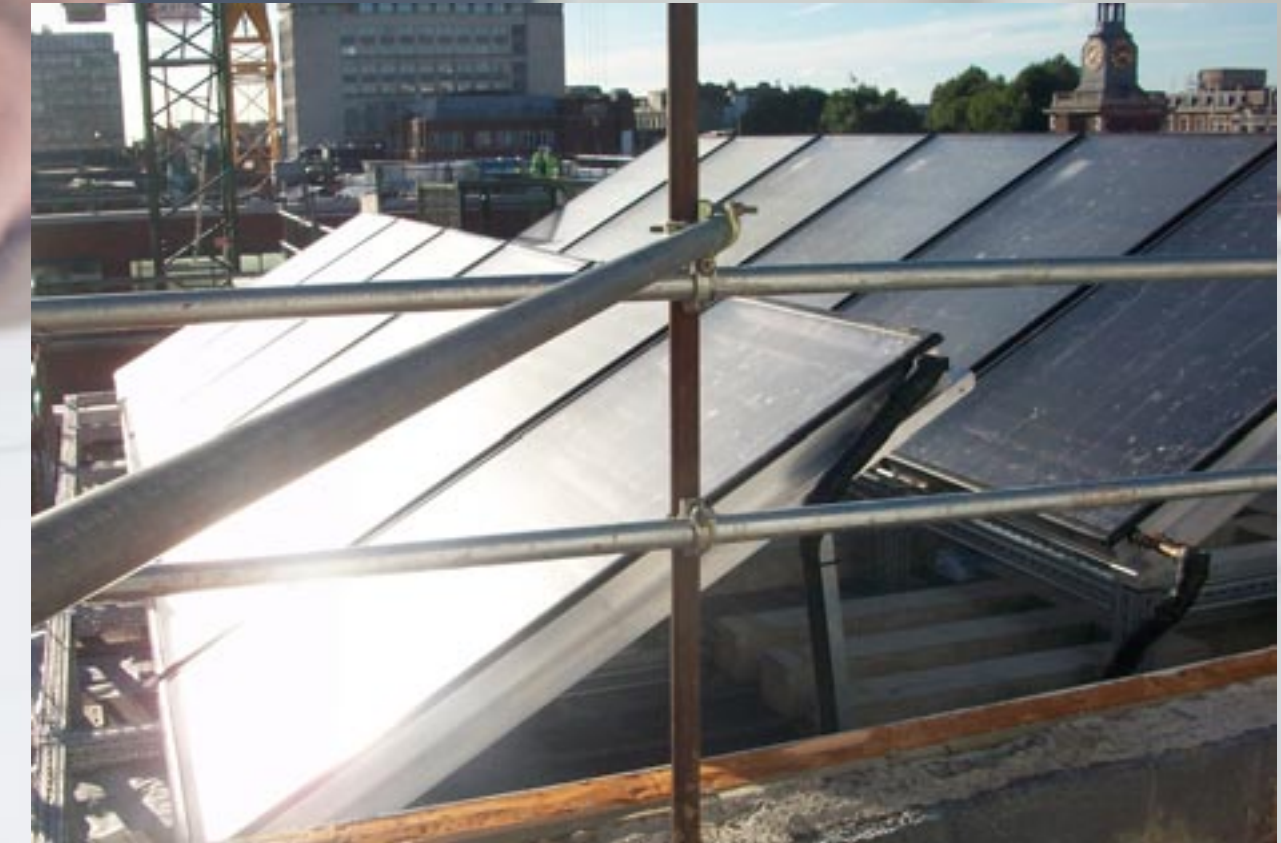
Solar thermal panels, London
