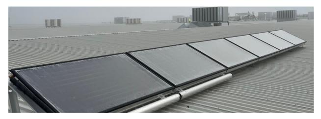
Adveco takes a look at the advantages of deploying solar thermal for hot water generation in commercial properties. As part of an organisation's wider sustainability plans, solar thermal offers a proven renewable technology that reduces emissions whilst able to integrate with other sustainable technology including air source heat pumps, direct electric and ultimately, through retained gas connections, hydrogen...
