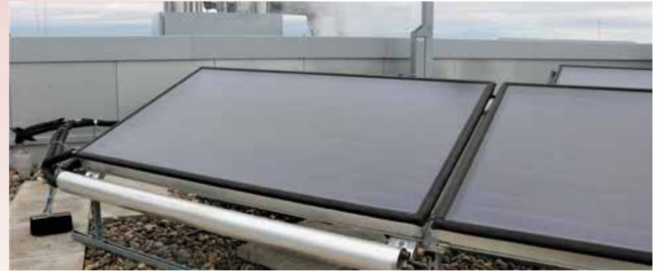
| Solar thermal preheat for gas-fired water heating
