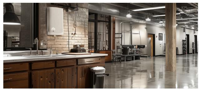
Point-of-use (POU) electric water heating in commercial applications was created for single outlet demands, usually far away from the plant room that would be difficult to supply in other ways. Typical examples of its application might be an outbuilding, very small buildings with low hot water demand, a tea point in a warehouse with few employees or a small washroom at the end of a long, dead-end corridor.
